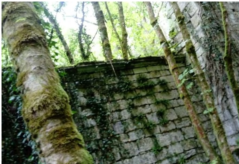
Figure 31 : Mur A, photo Bérénice Rondot, 2017.
